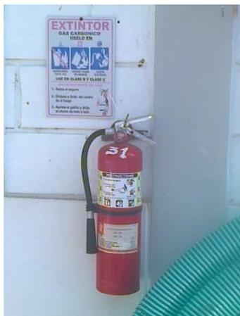
**FIG.25 Extintor CO<sub>2</sub>**
